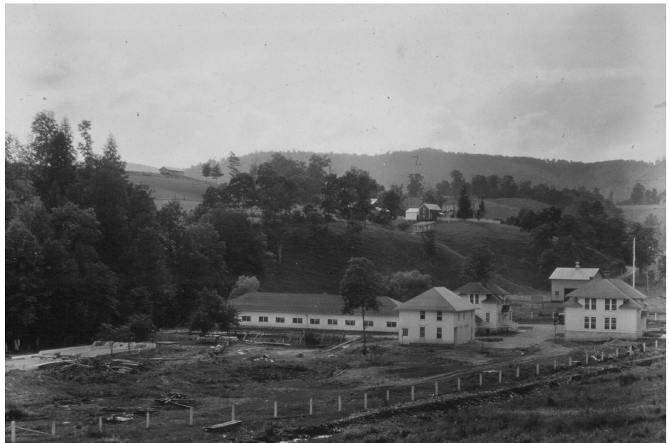
Edray Hatchery additional construction in 1935.
