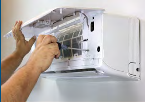
Back out electrical panel screws
