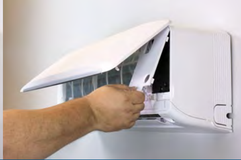
Remove electrical access panels (2)
