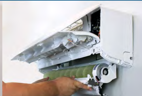
Remove screws then slide out the blower wheel assembly
