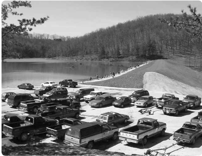
The Teter Creek Lake access site was developed with funds from the Sport Fish Restoration Program.
